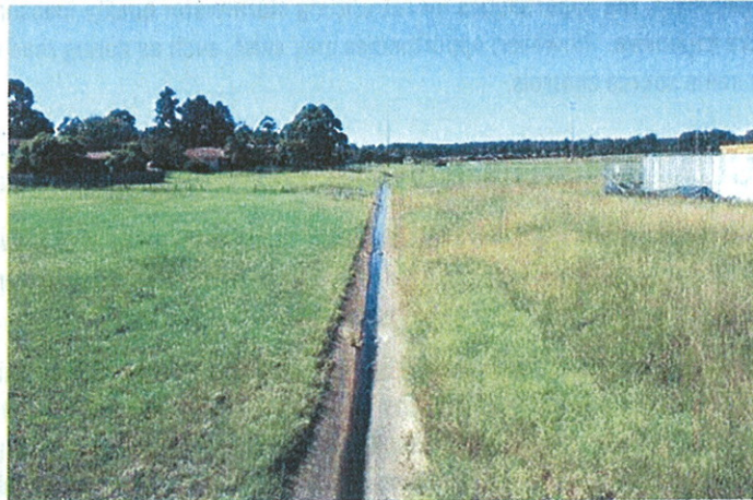
Plate 5: Concrete Lined Drainage Channel in Rosemeadow Reserve
