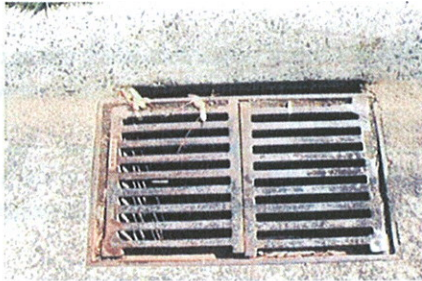
Plate 5: Typical Stormwater Pit in Existing Road
